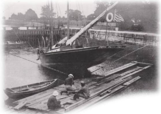
Schooner West Wing from Buffalo being repaired in Port Maitland Lock
