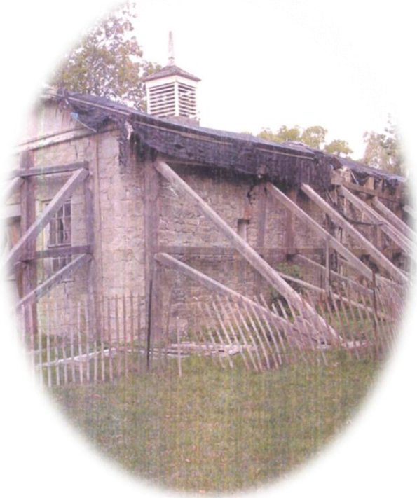
The Coach House prior to being rehabilitated/conserved.
