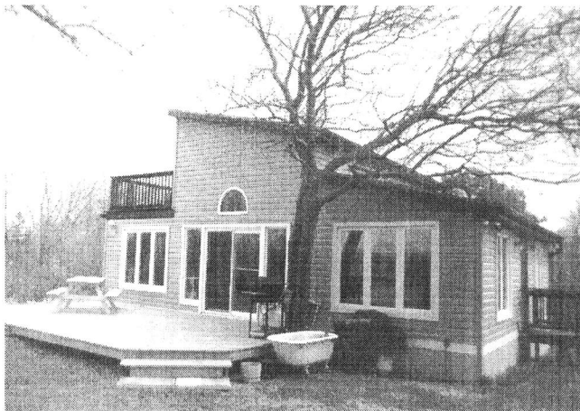
Recently rebuilt cottage of Fathers Ron and Dave Côté (lot 39) April, 1999.
