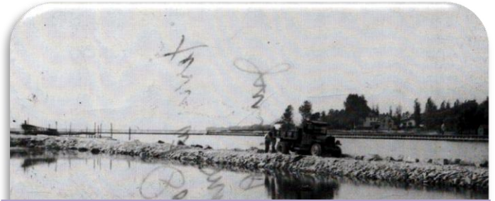
Placing of armour stone foundation in front of Hickey and Kelly cottages - October 11, 1937. Photo by Ed Boyle
