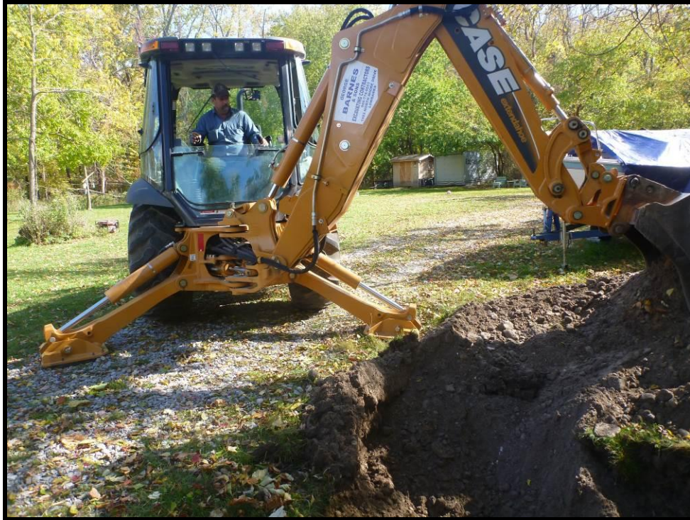
Image 13: View of Mechanical Excavation (Photo Taken on October 15, 2012; Facing Southeast)
