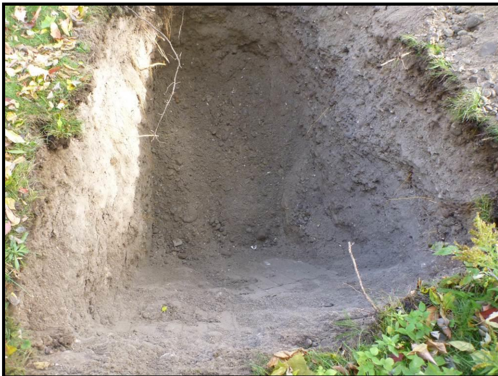
Image 14: View of Mechanical Excavation (Photo Taken on October 15, 2012; Facing Southeast)
